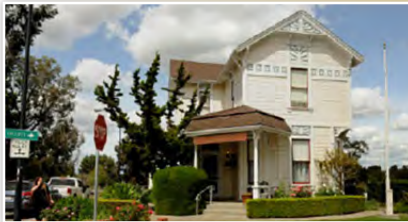
The Borland House is located across the street from the current District Office location.
